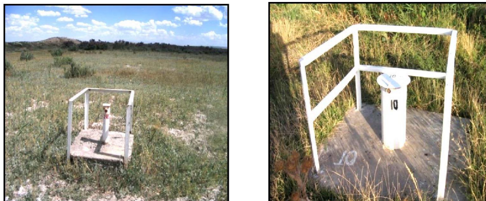
Figure 2 – Pictures of central and observation wells No. 261, 10
