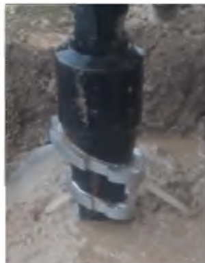
Figure 5 – Drilling process at low speeds of the drilling tool
