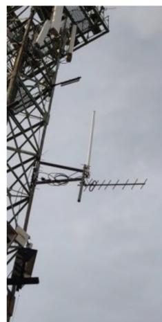
Figure 1 – VHF antennas of the BSDC transmitting complex on the Control's room antenna mast
