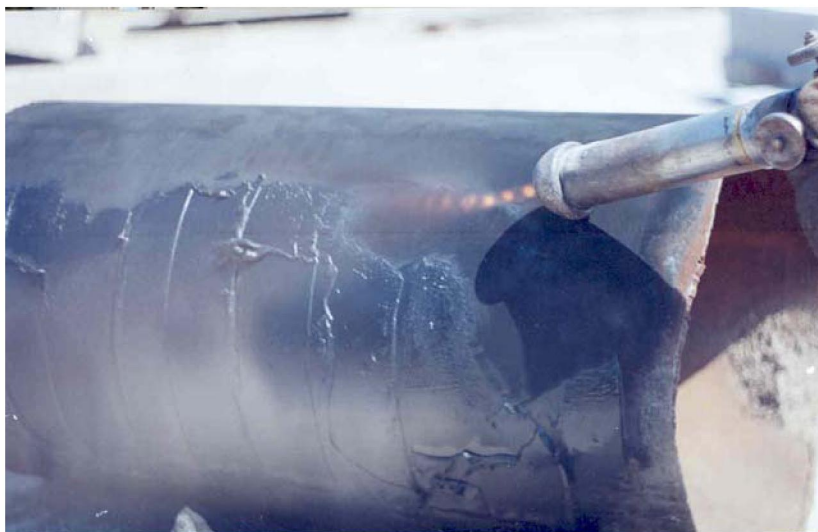
Figure 5 – Treatment of the pipe with a thermal hand-tool
