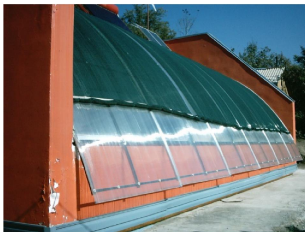
Photo 6 - Transparent fencing insulation of the experimental greenhouse from outside
